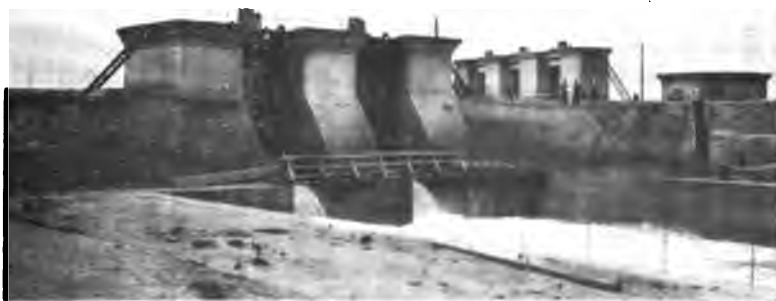
FIG. 101. —Headworks of Sultan Yab Canal at Sultan Bend Reservoir, on Murgab River, Turkestan.
